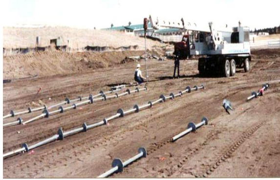
Photo 1-80 Hydraulic excavator installing helical piles for new commercial construction.
