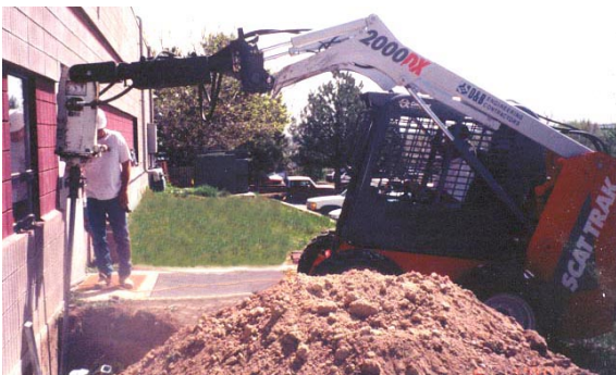
Photo 1-63 Skid-steer machine installing helical piles for foundation underpinning.
