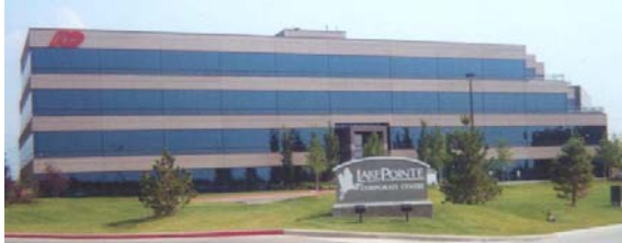
Photo 1-5 New multiple-story commercial structure designed and constructed on helical piles.
