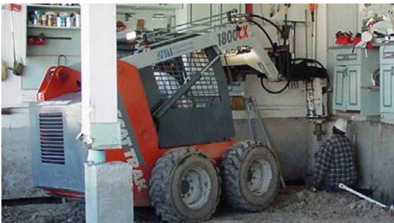
Photo 1-61 Skid-steer machine inside garage installing helical piles for foundation underpinning.
