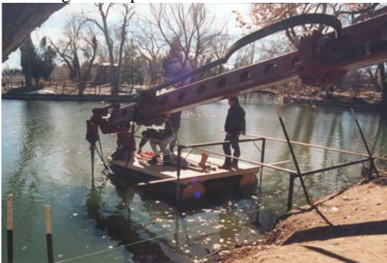
Photo 1-89 Hydraulic excavator boom mounted torque motor installing helical piles in lake.
