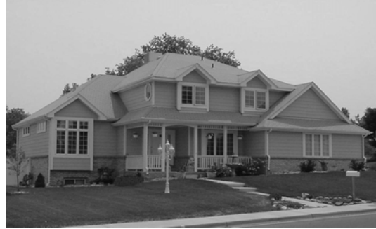
Photo 9-4 Residential struct. on helicals.
