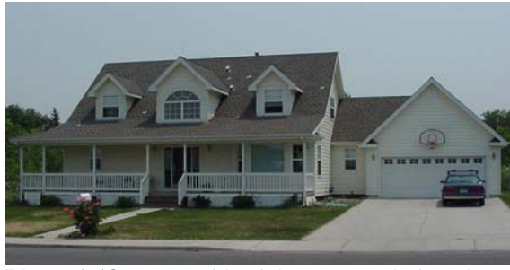
Photo 1-18 New residential structure designed and constructed on helical piles.
