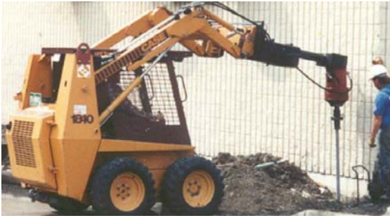
Photo 1-57 Skid-steer machine installing helical piles for foundation underpinning.
