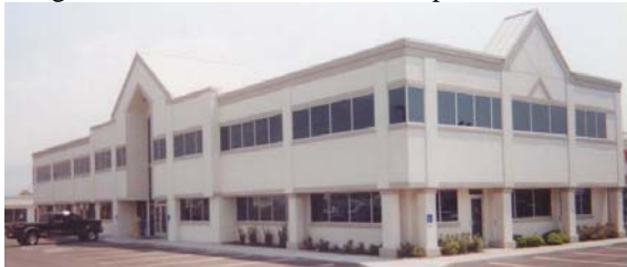
Photo 1-7 New office building designed and constructed on helical piles.
