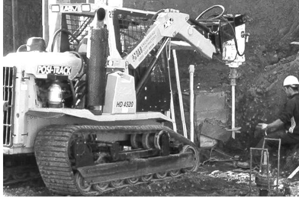
[Paper No. 2] Figure 6. Square Shaft Helical Pier Installation. 8,500 lb (38 kN) Machine
