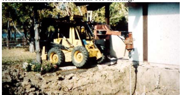
Photo 1-94 Skid-steer mounted torque motor installing helical piles for a new addition.
