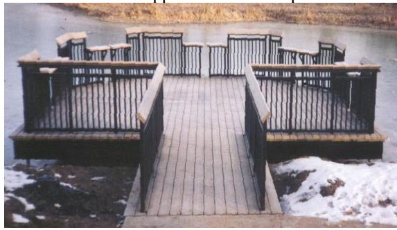
Photo 1-40 New fishing pier supported on helical piles.
