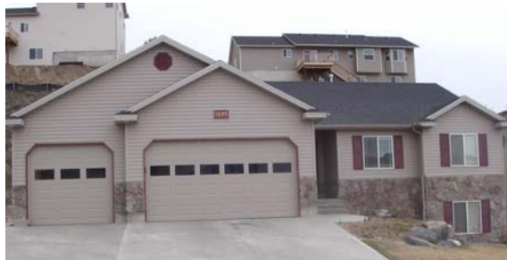
Photo 1-26 Existing residence with settled foundation underpinned/stabilized with helical piles.
