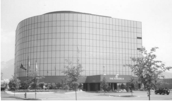
Photo 9-3 Multiple-story bldg on helicals.
