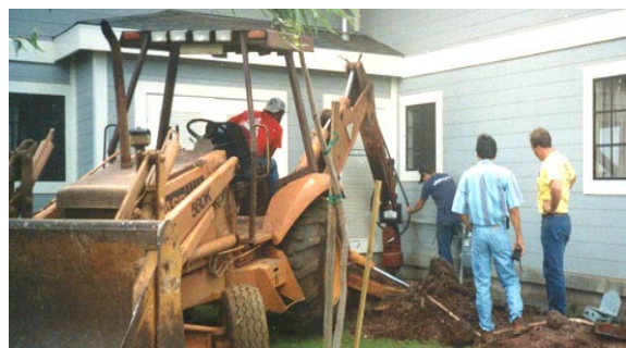
Photo 1-62 Backhoe installing helical piles for foundation underpinning.
