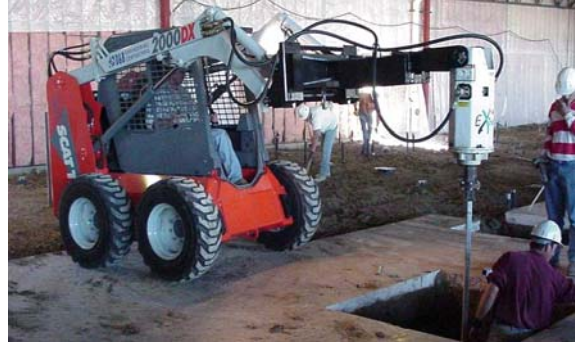
Photo 1-64 Skid-steer machine inside a building installing helical piles for foundation retro-fit.
