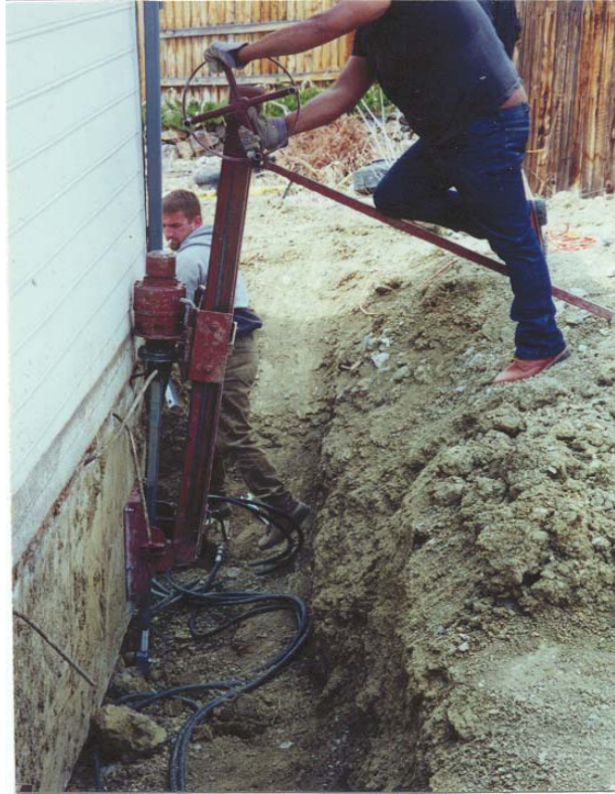
Photo 1-66 Hand-carried mast for installation of helical piles in tight access location.
