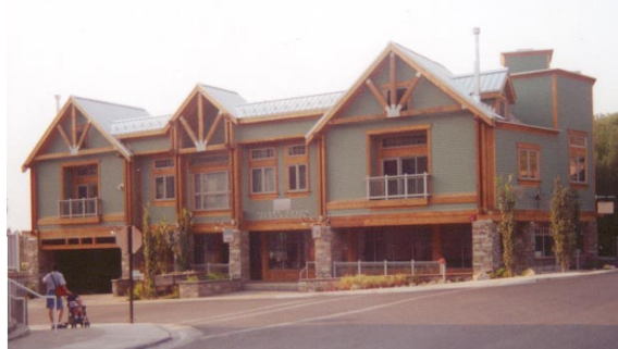
Photo 1-22 New residential condominium structure designed and built on helical piles.
