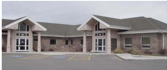
Photo 1-30 Existing building with settled foundation underpinned and stabilized with helical piles.
