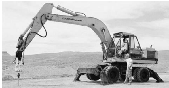
[Paper No. 2] Figure 2. Square Shaft Helical Pier Installation Using a Wheeled Hydraulic Excavator
