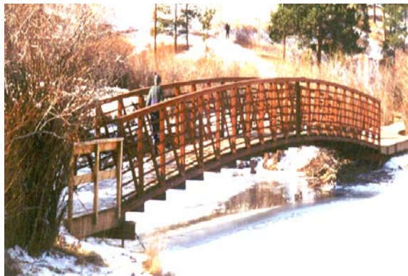
Photo 1-36 New pedestrian bridge with abutments supported on helical piles.
