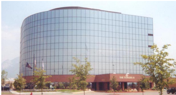
Photo 1-1 New multiple-story commercial structure designed and constructed on helical piles.
