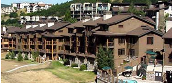
Photo 1-3 New condominium structure in a resort area designed and constructed on helical piles.
