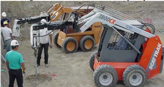
Photo 1-55 Skid-steer type machines installing helical piles for new construction.
