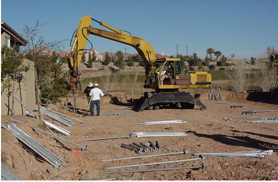
Photo 1-79 Hydraulic excavator installing helical piles for new foundation.
