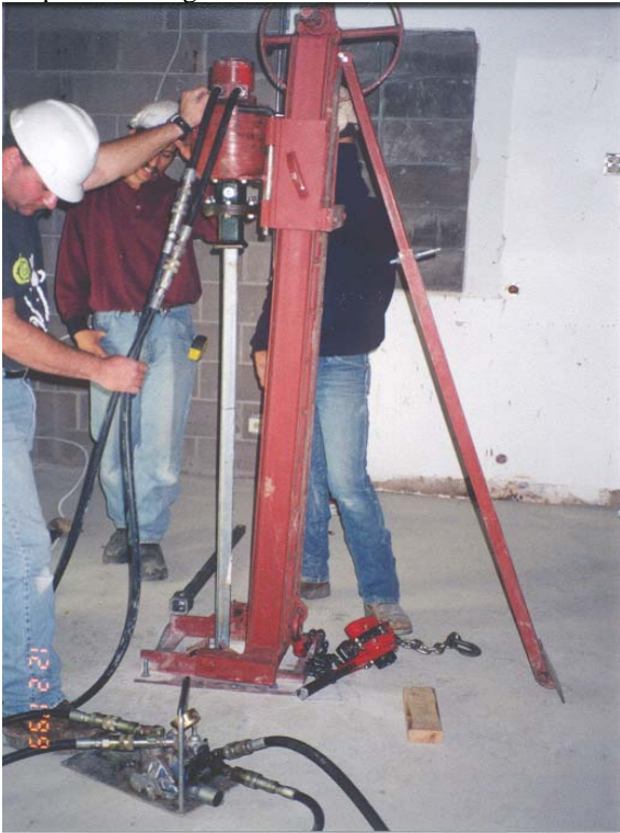
Photo 1-67 Hand-carried mast for installation of helical piles in tight access location.
