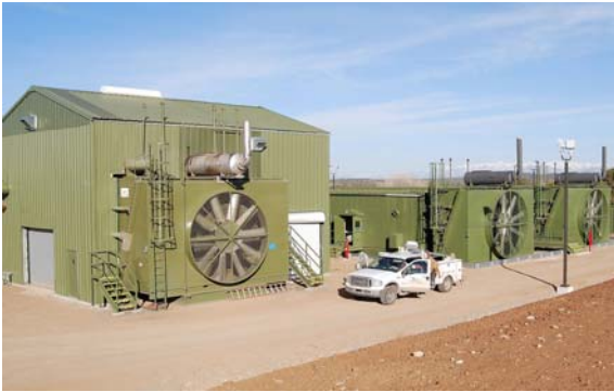
Photo 1-9 New natural gas compressor station designed and constructed on helical piles.
