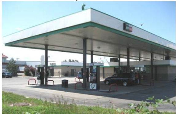
Photo 1-14 New gas pump facility. All structures designed and constructed on helical piles.
