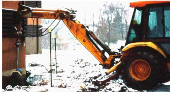
Photo 1-58 Backhoe installing helical piles for foundation underpinning.
