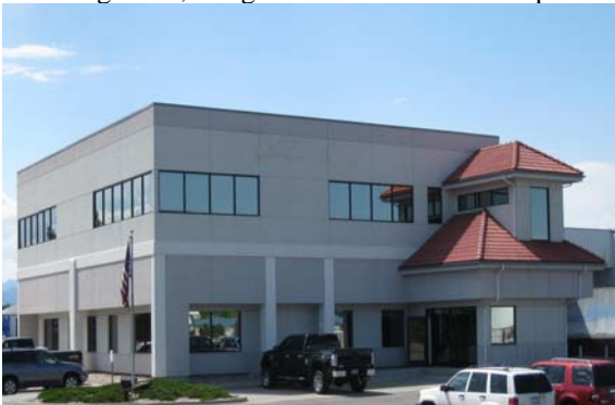
Photo 1-13 New office building designed and constructed on helical piles.
