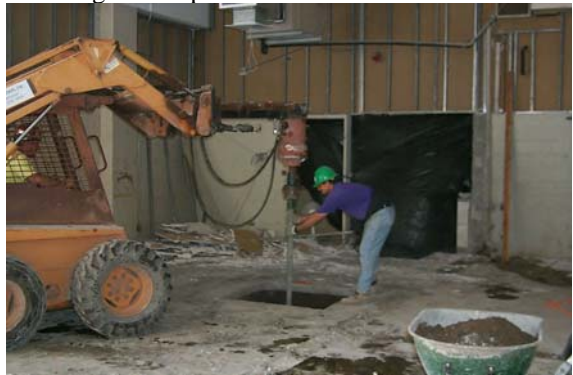
Photo 1-90 Skid-steer mounted torque motor installing helical piles inside existing building.
