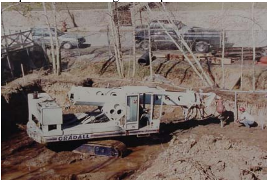
Photo 1-91 Hydraulic excavator mounted torque motor installing helical piles.
