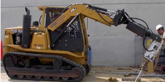
Photo 1-83 Tracked machine installing battered helical piles for lateral load resistance.
