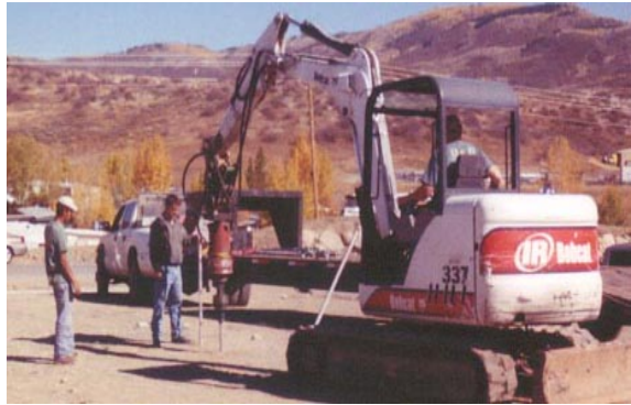
Photo 1-88 Mini-excavator mounted torque motor installing helical piles.
