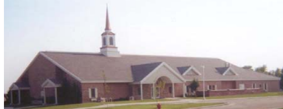
Photo 1-6 New church building designed and constructed on helical piles.
