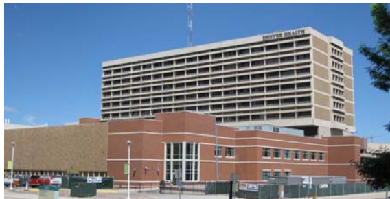
Photo 1-28 The existing nine-story structure was underpinned and shored with helical piles.
