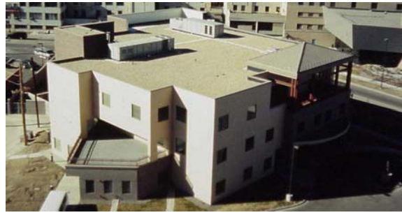
Photo 1-2 New multiple-story commercial structure designed and constructed on helical piles.
