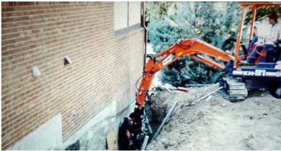
Photo 1-59 Mini-excavator installing helical piles for foundation underpin.
