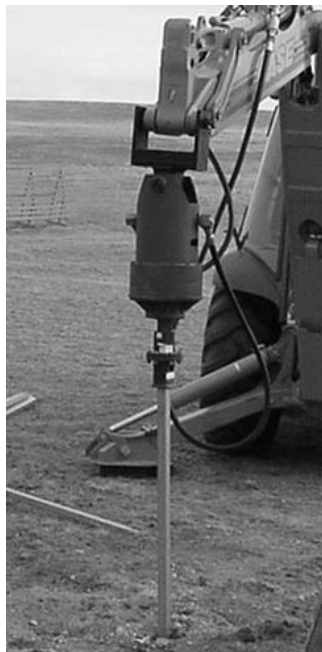
Photo 9-1 Installation with hydraulic drive head mounted on a backhoe boom.
