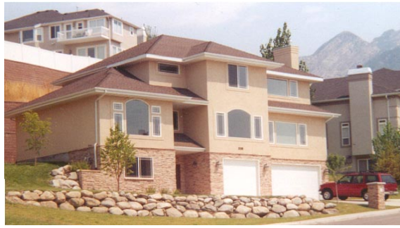
Photo 1-20 New residential structure designed and constructed on helical piles.
