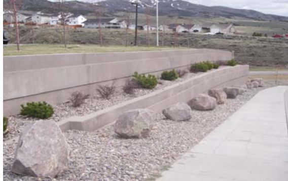
Photo 1-42 New reinforced concrete retaining wall using helical tension anchors as tiebacks.
