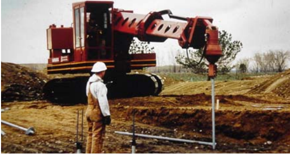
Photo 1-49 Tracked hydraulic excavator capable of installing over 60 helical piles per day.
