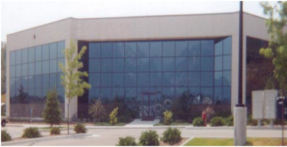
Photo 1-25 Existing building with settled foundation underpinned and stabilized with helical piles.
