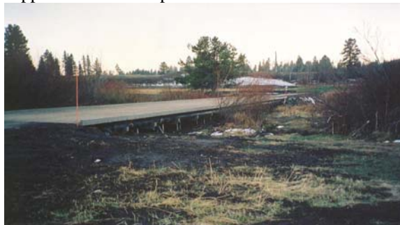
Photo 1-38 New golf cart/pedestrian/vehicle bridge in marsh wetland supported on helical piles.
