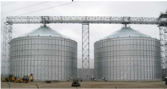
Photo 1-15 New large grain elevator facility designed and constructed on helical piles.
