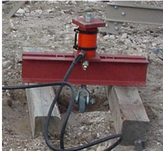
Photo 3-2 Tension load test set-up for Helical Tension Anchor.
