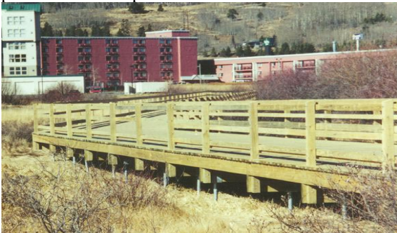
Photo 1-39 New boardwalk in marsh wetland supported on helical piles.
