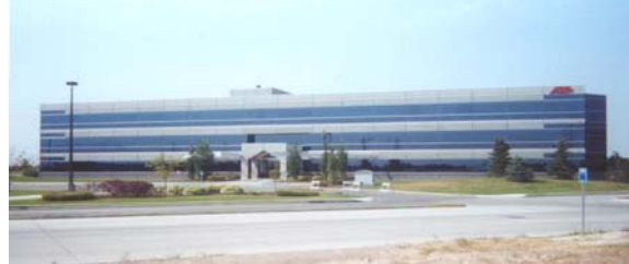
Photo 1-8 New multiple-story commercial structure designed and constructed on helical piles.
