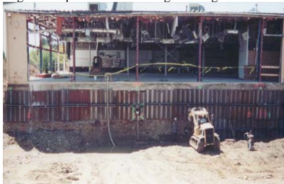
Photo 1-92 Tracked machine installing helical tension anchors as tiebacks for shoring.
