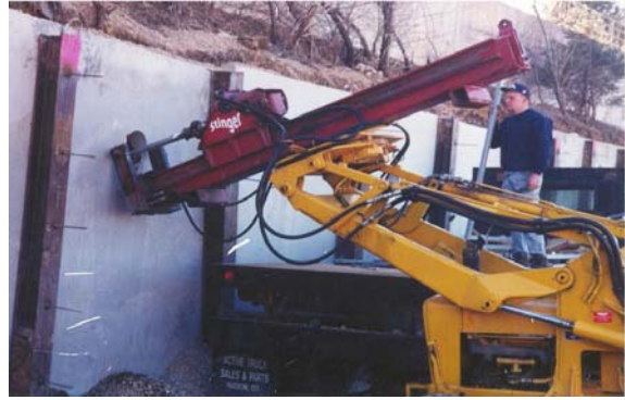
Photo 1-72 Loader mounted torque motor installing helical tension anchors as tiebacks for repair.
