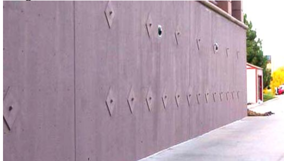
Photo 1-46 Existing foundation/retaining wall laterally supported with helical anchors as tiebacks.
