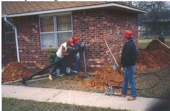
Photo 1-70 Hand-carried torque motor, yoke, and torque arm for tight access location.
