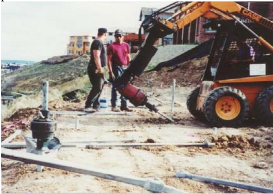
Photo 1-81 Skid-steer mounted torque motor installing battered helical tension anchor under itself.
