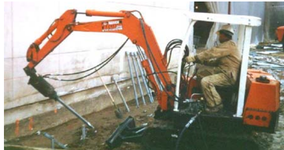
Photo 1-60 Mini-excavator installing battered helical piles adjacent to existing building.
