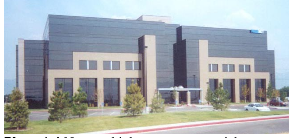
Photo 1-4 New multiple-story commercial structure designed and constructed on helical piles.
