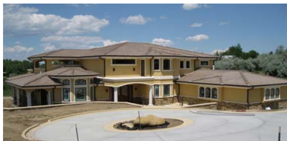
Photo 1-24 New residential structure designed and constructed on helical piles.
