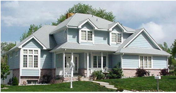
Photo 1-17 New residential structure designed and constructed on helical piles.
