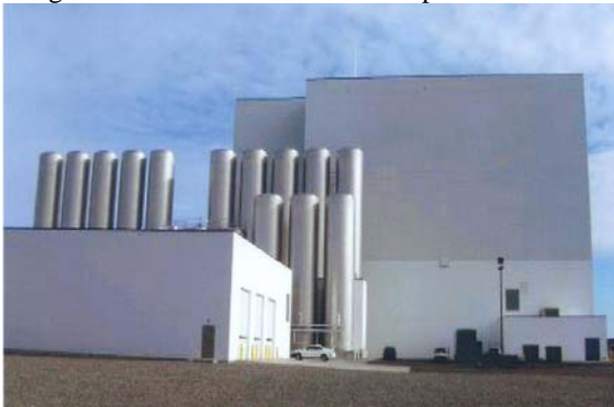
Photo 1-11 New Industrial facility, all structures, including tanks, designed and built on helical piles.
