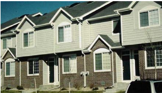
Photo 1-19 New residential condominium structure designed and constructed on helical piles.
