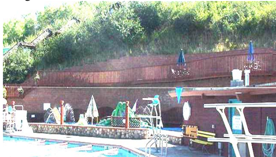
Photo 1-44 New reinforced concrete retaining wall using helical tension anchors as tiebacks.
