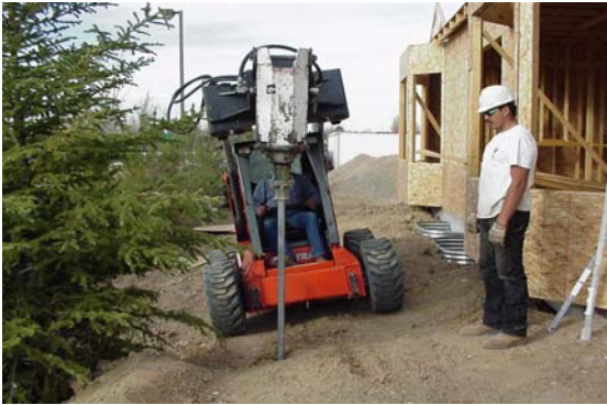
Photo 1-87 Skid-steer mounted torque motor installing helical piles.
