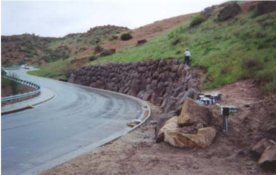
Photo 1-41 New rock faced retaining wall using helical tension anchors as tiebacks.
