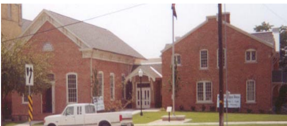
Photo 1-31 Existing rubble foundation under this historic structure replaced using helical piles.
