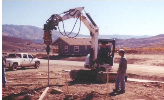
Photo 1-56 Mini-excavator is capable of installing over 60 helical piles per day.
