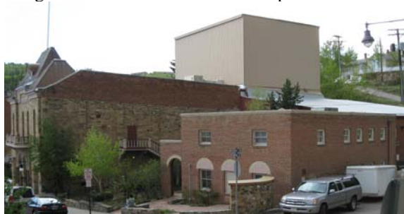
Photo 1-16 New annex to historical structure designed and constructed on helical piles.
