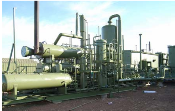
Photo 1-10 New natural gas facility designed and constructed on helical piles.
