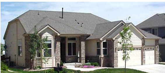
Photo 1-29 Existing residence with settle foundation underpinned and stabilized with helical piles.
