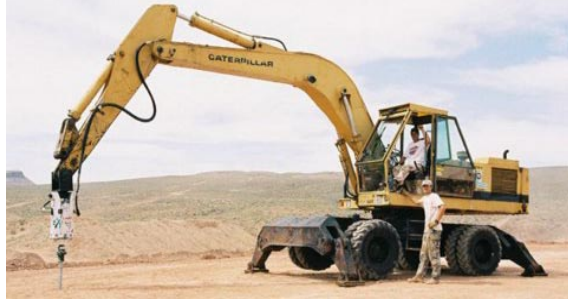
Photo 1-50 Rubber-tired hydraulic excavator capable of installing over 60 helical piles per day.
