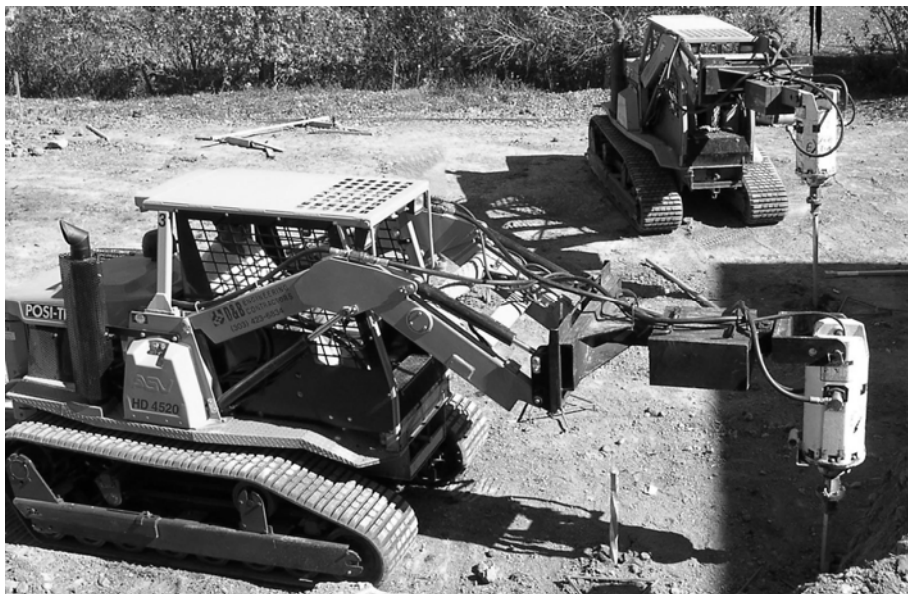
[Paper No. 1] Figure 2. Square Shaft Helical Pier Installation.
