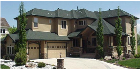
Photo 1-23 New residential structure designed and constructed on helical piles.
