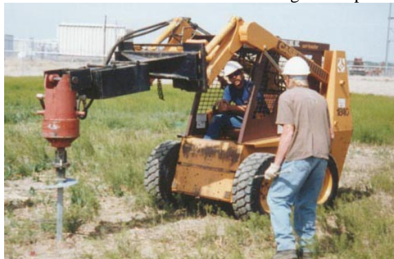
Photo 1-86 Skid-steer mounted torque motor installing helical screw piles.
