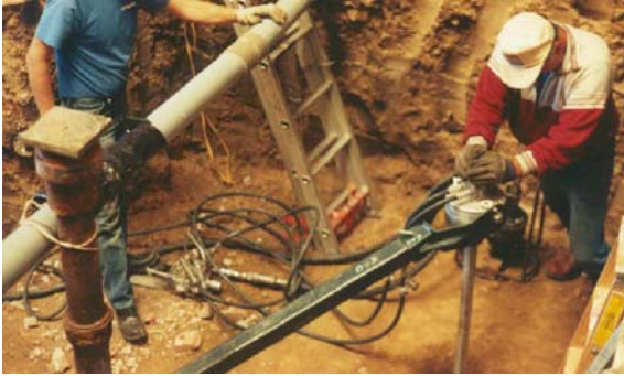
Photo 1-65 Hand-carried torque motor, yoke, and torque arm in tight access location.
