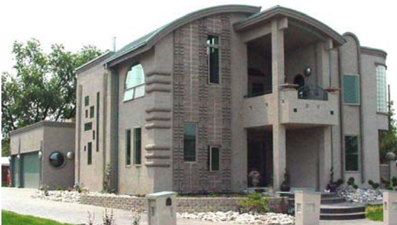
Photo 1-21 New residential structure designed and constructed on helical piles.
