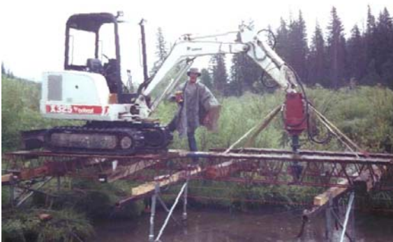
Photo 1-85 Mini-excavator mounted torque motor installing helical screw piles over wetland.
