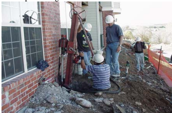
Photo 1-68 Hand-carried mast for installation of helical piles in tight access location.
