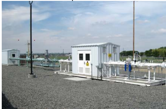
Photo 1-12 New natural gas facility designed and constructed on helical piles.
