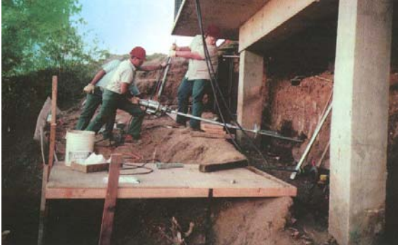
Photo 1-77 Hand-carried equipment installing helical tension anchors as tiebacks for repair.
